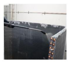
1. Spray the coil with water and a non-acidic detergent (ex: dish soap) in a side-to-side motion starting at the top
