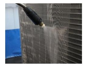
(Proper Angle to avoid damage to the coil)
