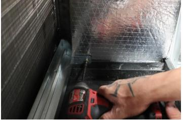
3. Install Bottom and Side Filter Rack and (A, B + C, D)
