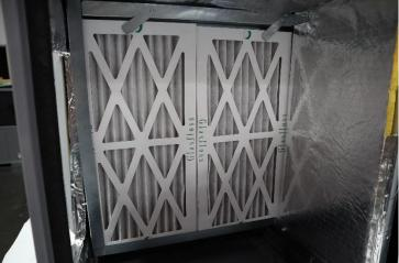
4. Install Filters (H) and secure them using the Filter Latches (G)
