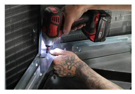
6. Screw the Filter Rack Center (E) to the bottom Filter Rack Assembly (A + B1 + B2)
